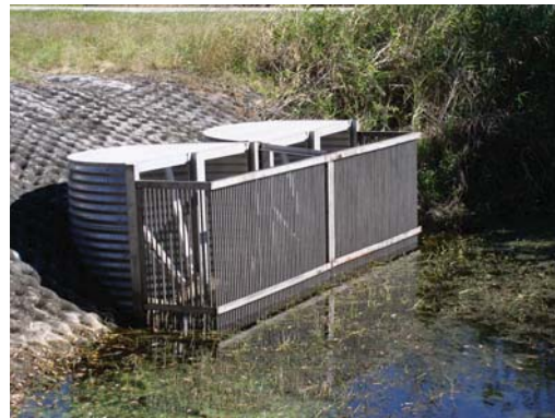
Figure 2. Fish Fence installed on outlet to Lake June
